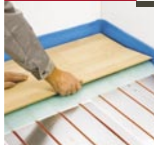
Installation of the wooden floor
