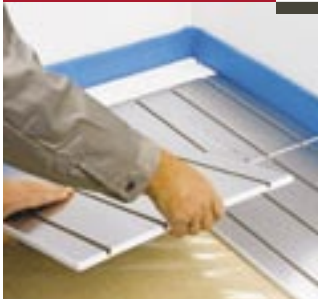
Installation of plates
