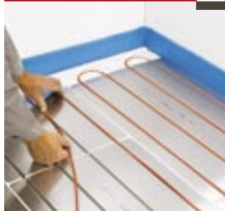
Install heating cable
