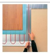
T2Reflecta and T2Red floor heating system consists of an insulated aluminium profile T2Reflecta and the self-regulating T2Red heating cable
